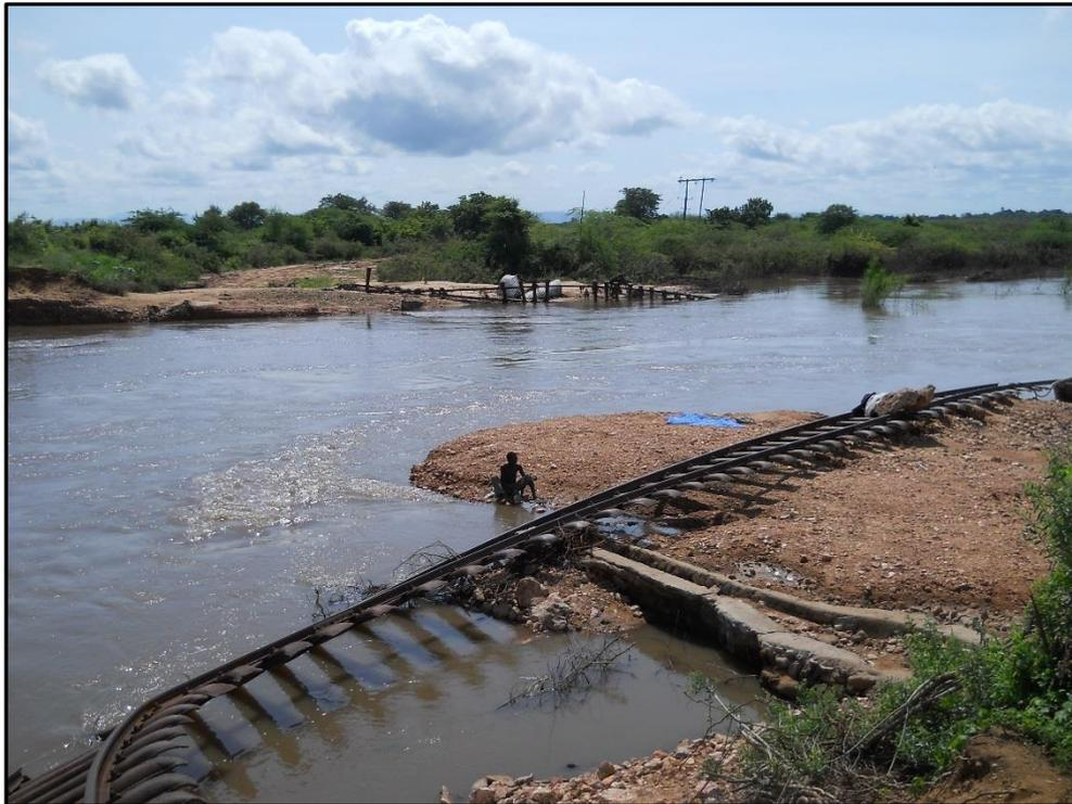
**Figure 2.13** Collapse of the rail line caused by breaching and washaway of the supporting embankment
