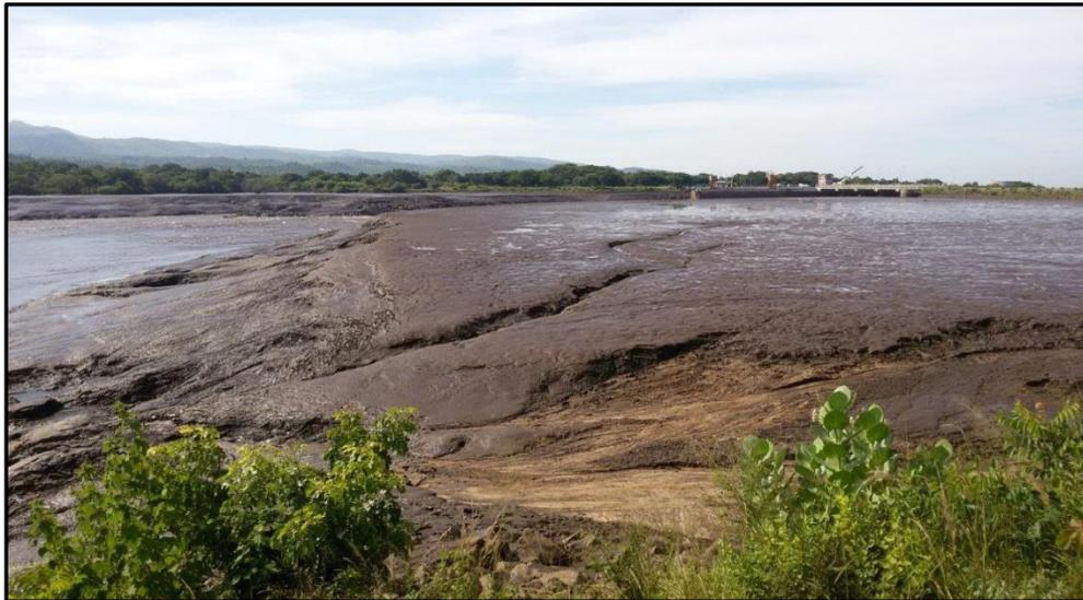
**Figure 6.4** Siltation of the Kapachira Reservoir, exposed during ‘desilting’ in March 2016; photograph taken looking downstream towards the dam wall on the far-right
