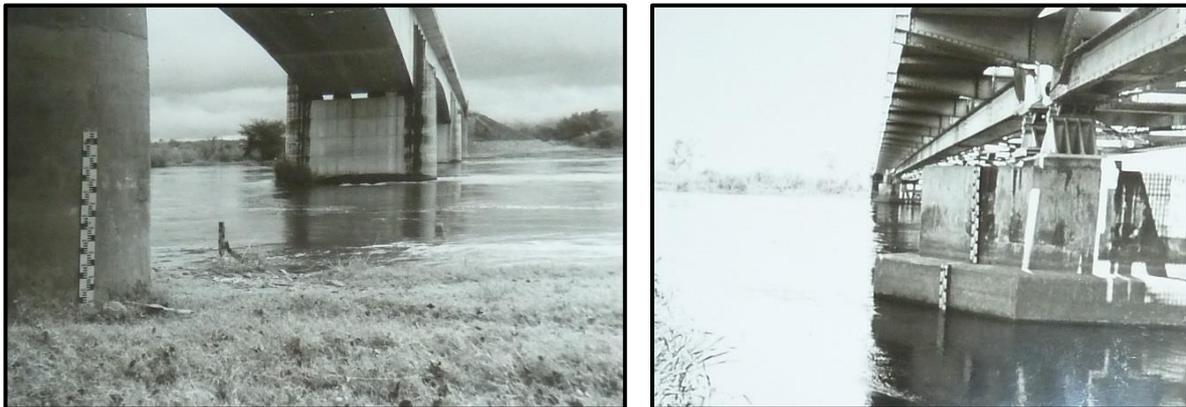
**Figure 3.5** Historic photographs<sup>132</sup> of gauge stations with plates fixed to bridge piers, left: Chikwawa (1L12) located at the Kamuzu Bridge (1979), and right: Chiromo (1G1) at the railway bridge (undated, circa 1970/80s)
